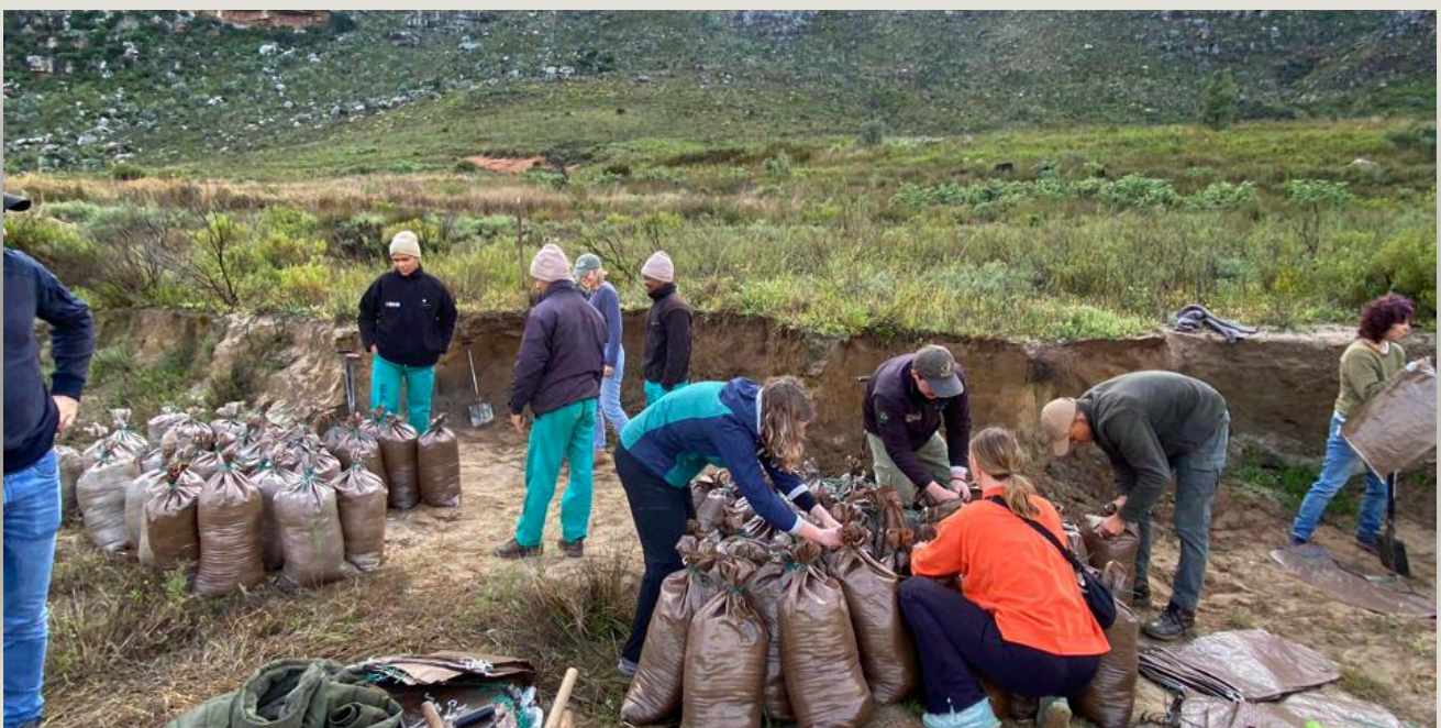
Fig 5: Volunteers and CapeNature personnel filling sandbags to help prevent further erosion.
